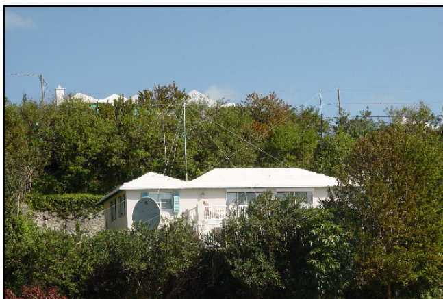
View from road at base of hill, south of the house.
