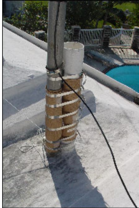
Base of the mast for the beam. The rubber sheeting is to prevent the mast from rotating
