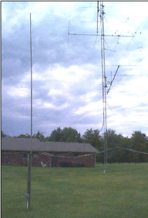
The array consists of eight short verticals (21') in a circle with a diameter of 350'.
