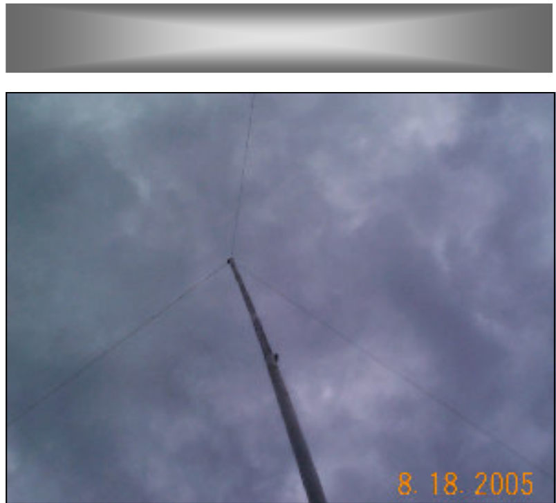
There are three top hat wires about 33' long and three buried radials under each one.
