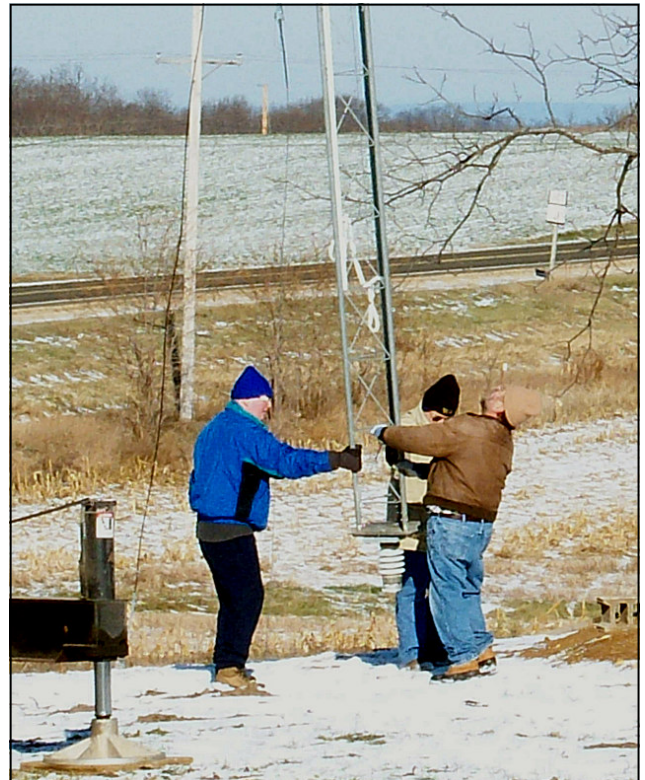
W19WI, K9AY and K9MA guide the tower onto the pier pin base. The base insulator (courtesy of W0AIH) has no problem supporting this light tower. We're dressed for the cold, but it was really quite nice WX at 40F, bright sunshine and minimal wind.
