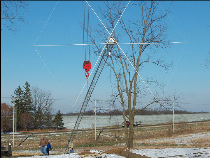
100 ft. of Rohn 25G stayed pretty straight when lifted at the 70-foot point. This photo provides a good look at the capacity hat on this tower.
