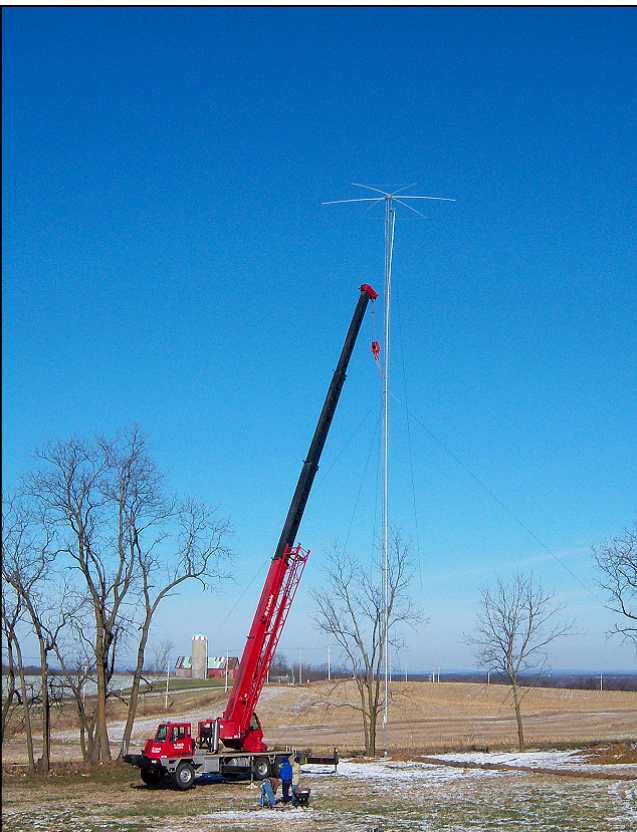
We're tensioning the last guy wire before I climbed the tower to unhook the lifting sling and let the crane leave. This is the view from my driveway toward the north.
